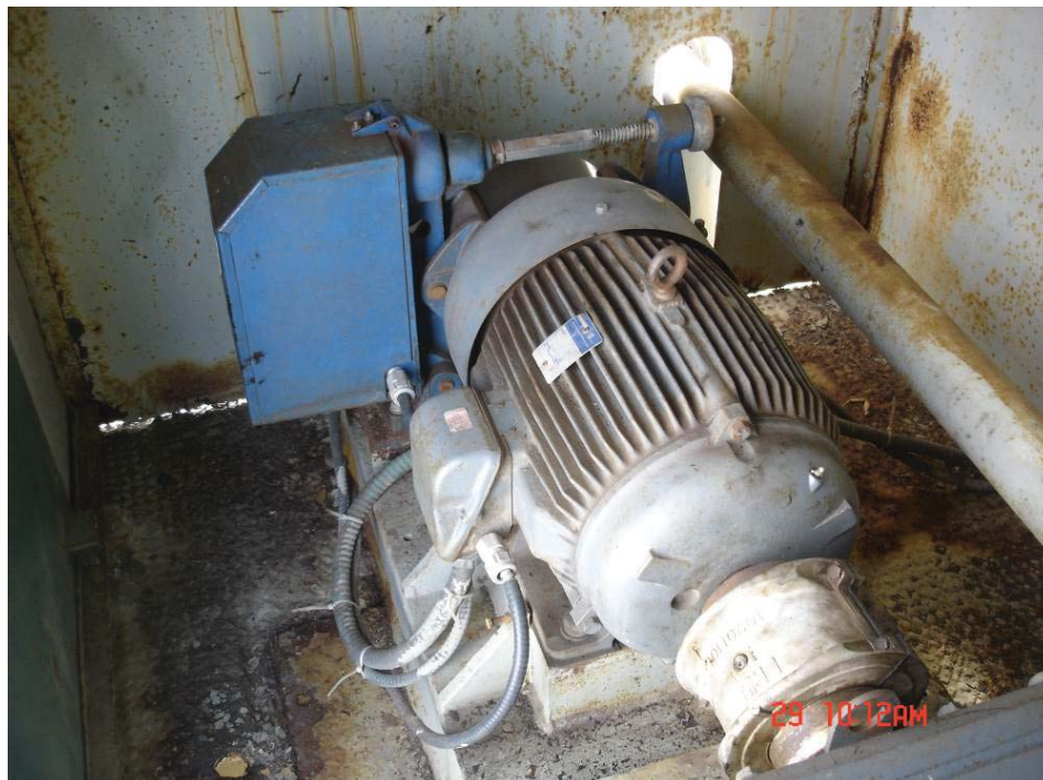
Photo 12 – Perigrip Brake on the Back Side of the Hoist Motor
