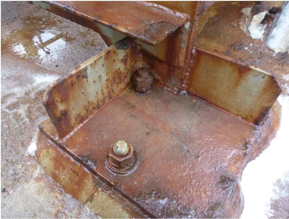
Photo 1 – Typical Tower Base Plates
