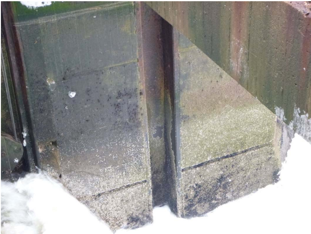
Photo 6 – Stoplog Guides (Tidal Side)
