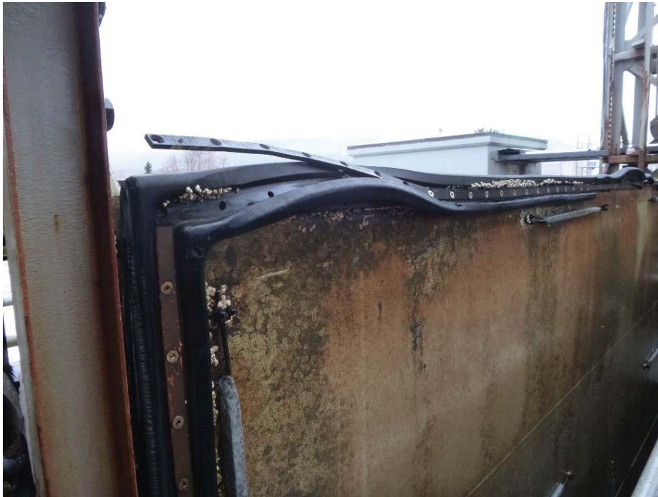
Photo 6 – Spillway Gate #2 Lintel Seal
