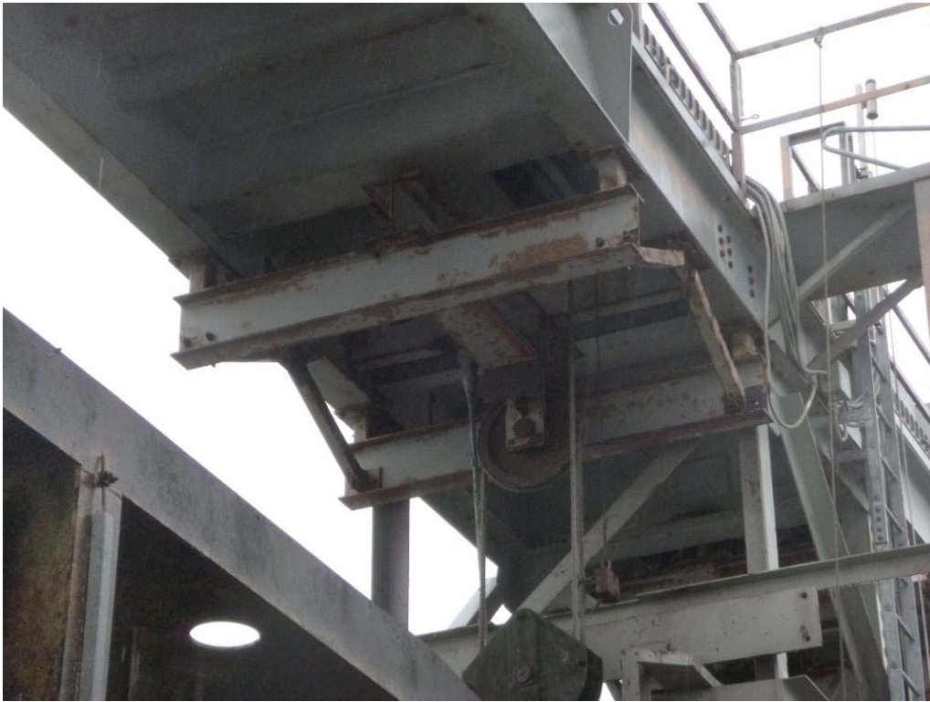
Photo 5 – Upper Sheave Support Suspended Structure
