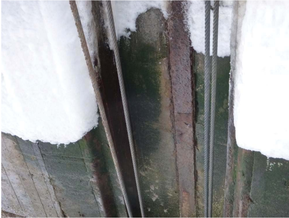
Photo 3 – Gate Guide Side Roller Path
