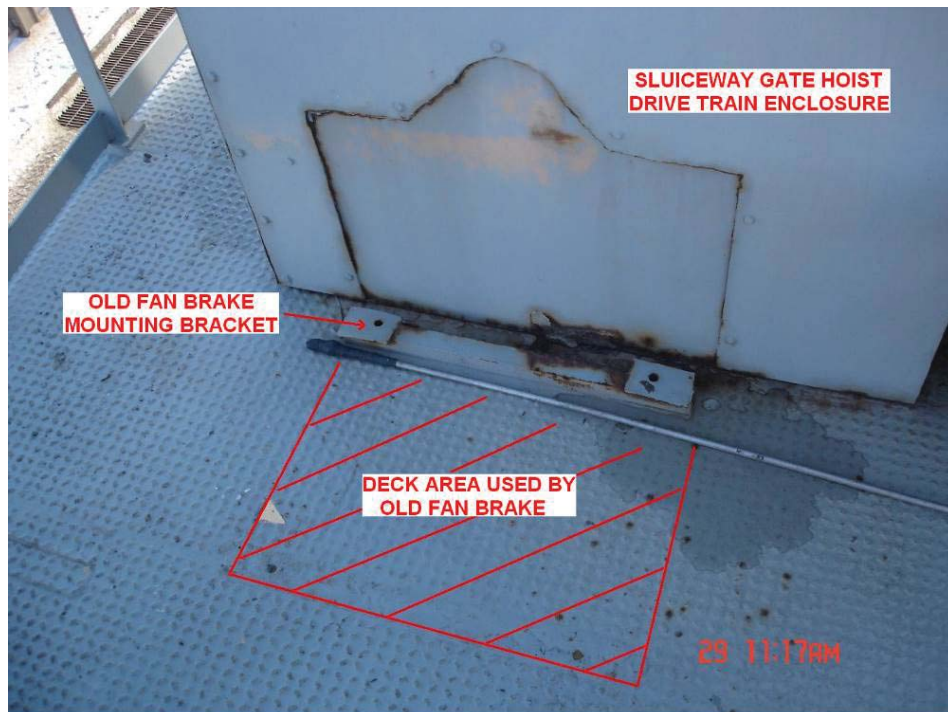
Photo 10 – Exterior of Sluiceway Gate Hoist Drive Train Enclosure
