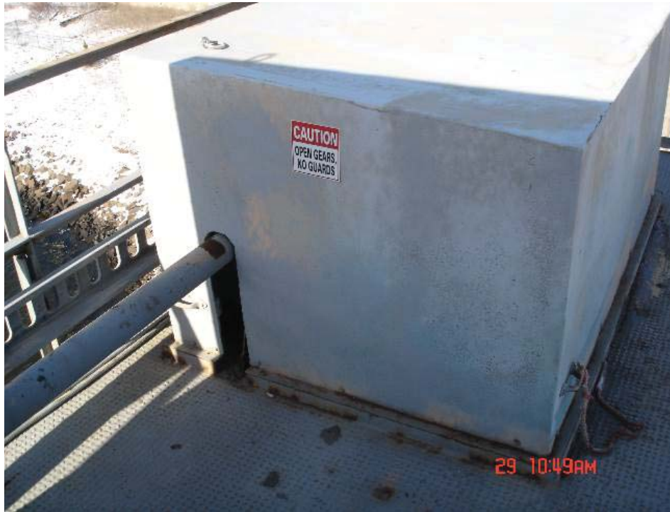
Photo 17 – Drive Shaft Enclosure
