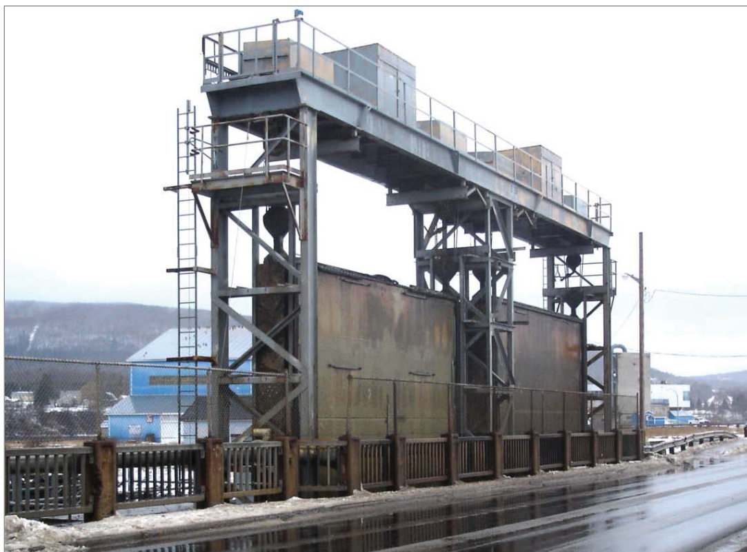
Photo 2 – Annapolis Sluiceway Gates and Superstructure
