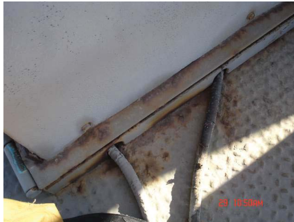
Photo 20 – Electrical Conduit Penetration
