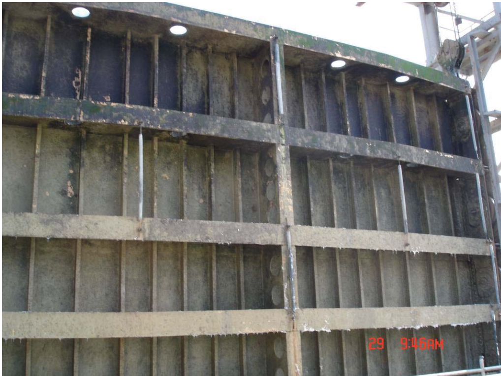
Photo 12 – Back (Tidal side) of Spillway Gate - Typical
