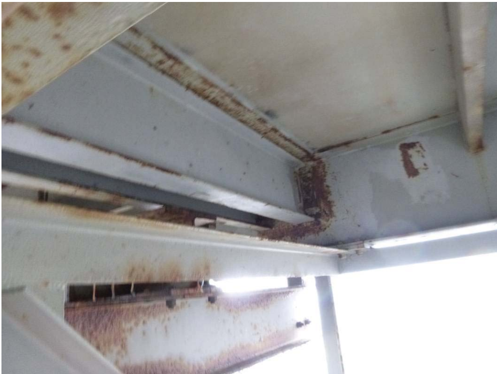
Photo 4 – Box Beam Replaced with S-beam and Channel – Bolted Connections
