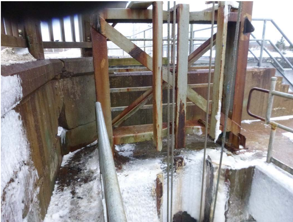
Photo 2 – Typical Surface Corrosion and Staining on Lower Portions of Towers
