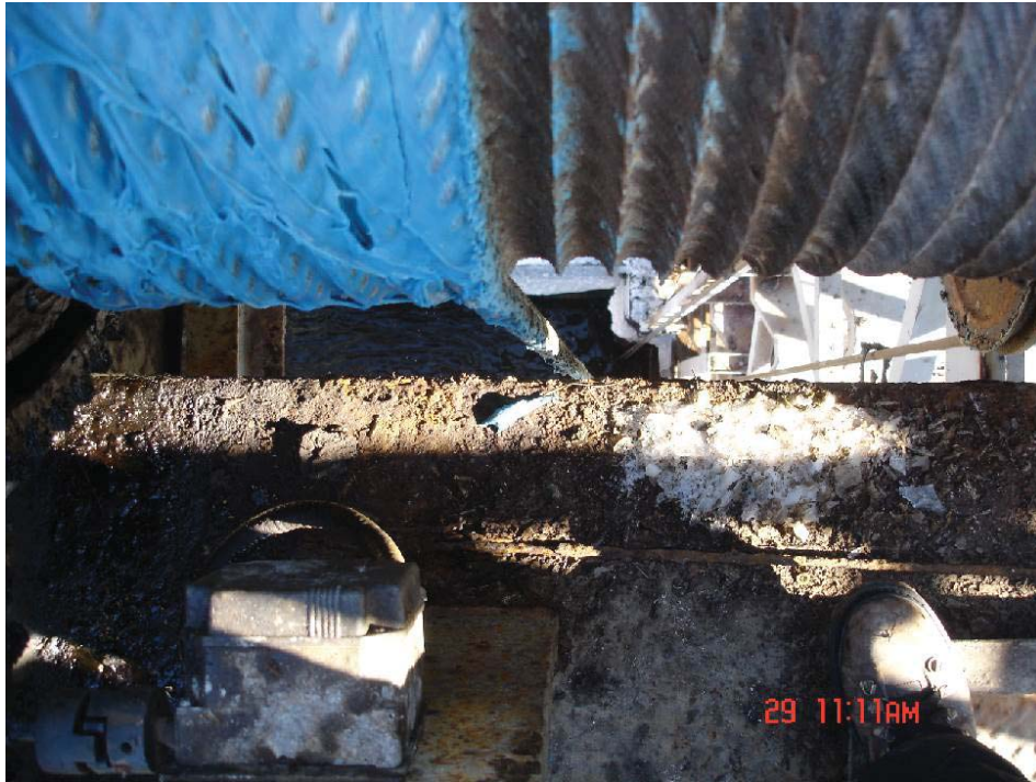
Photo 13 – Dynagard Blue on Hoist Wire Rope
