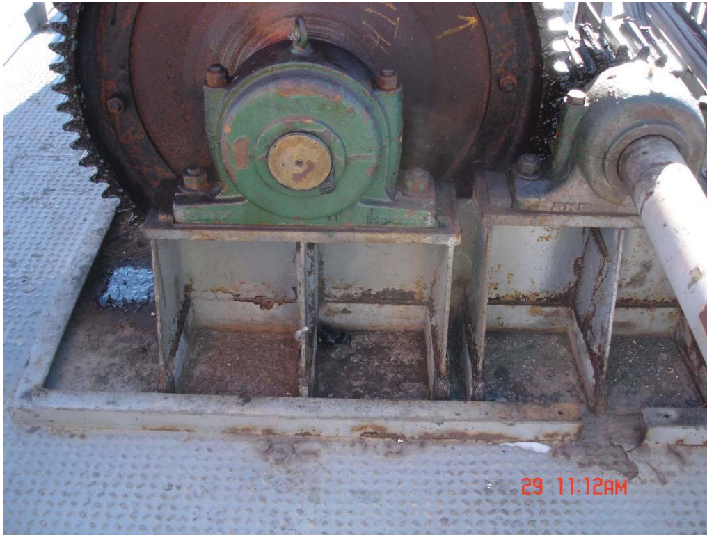
Photo 15 – Reinforcement Plates on Center Stiffeners
