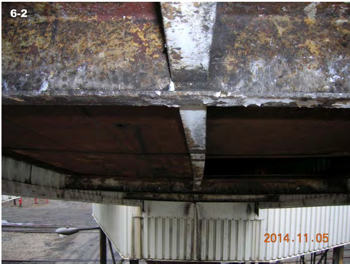
Longitudinal Channel Bowed out of Plane
