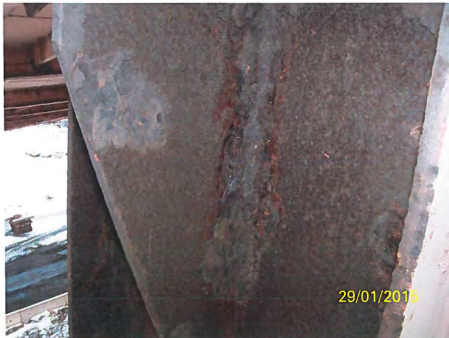
Photo 2a - Stiffener just below Bearing on West Side
