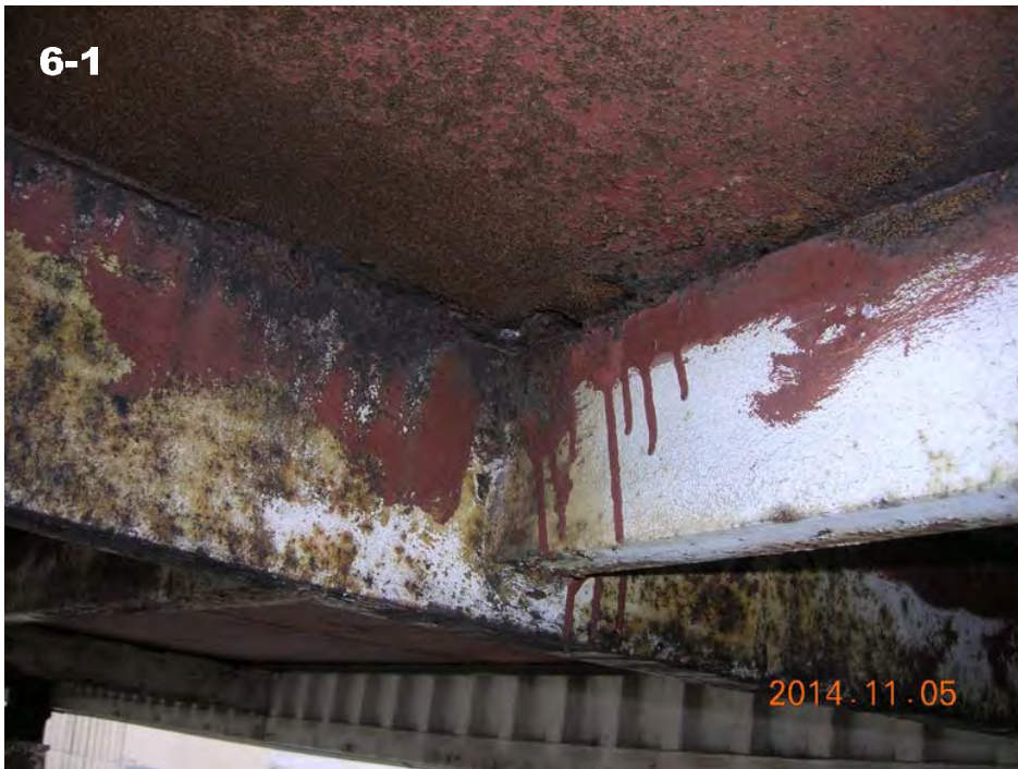
Attachment of 4" Longitudinal Channel to 5" Transverse Channel
