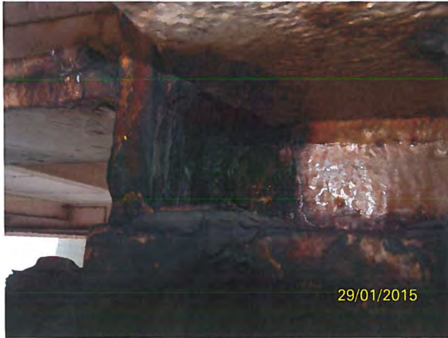
Photo 1b - West Side Bearing Viewed from the South
