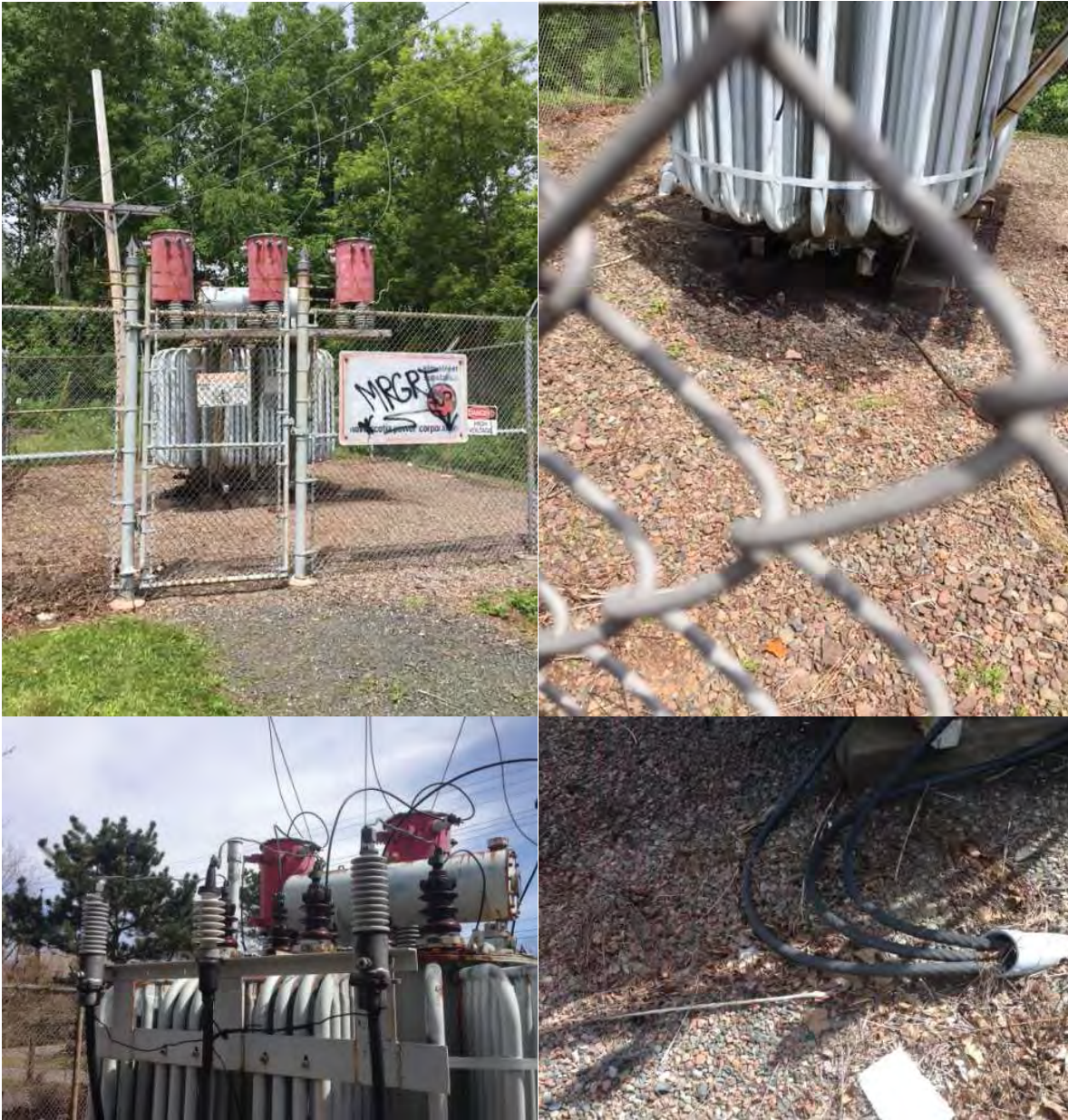
Figure 6 Photos of 532N-Elm St
