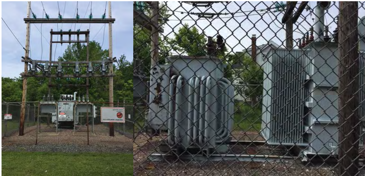
Figure 5 Photos of 528N-Granville St
