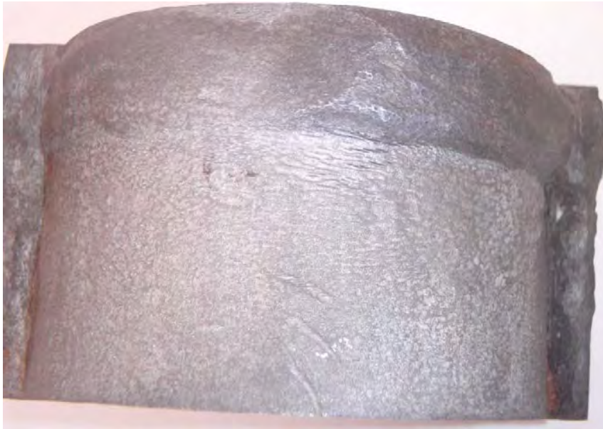
Photograph 25 Circumferential Cracks on Crown of Hot Side Exterior
