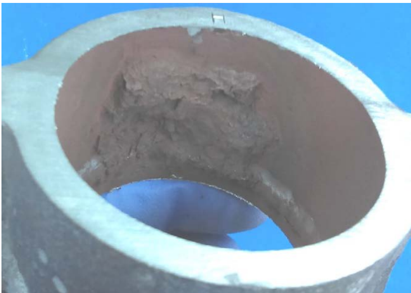
Photograph 1 Hot Side Before Cleaning
