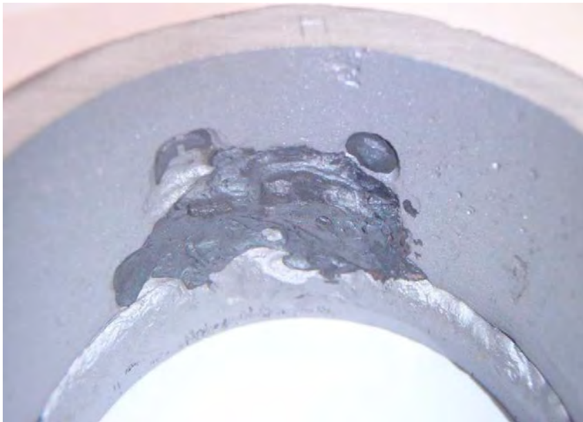
Photograph 24 Hot Side Surface After Bead Blasting
