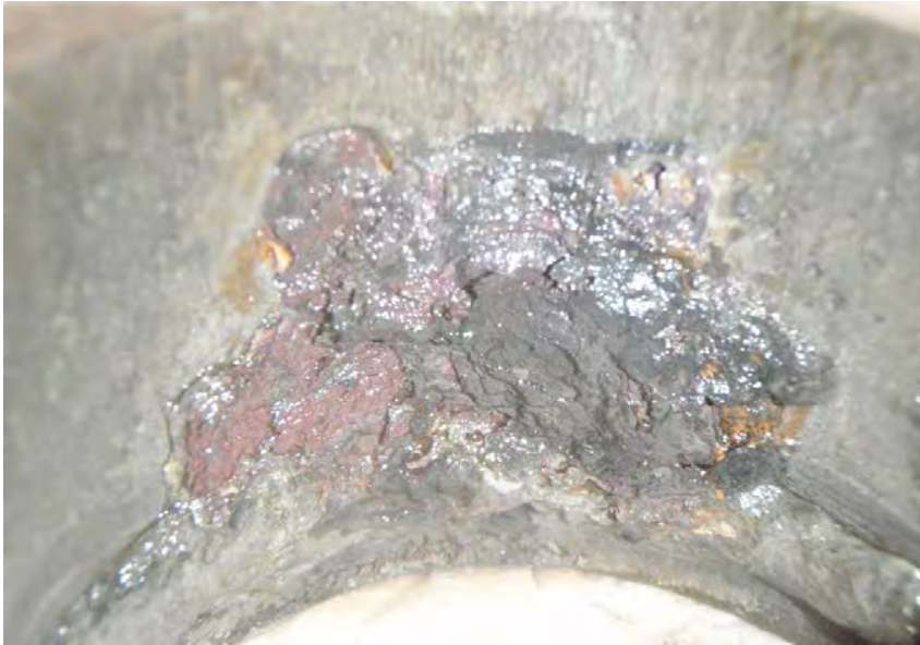
Photograph 19 After 4 th Stage (Final Copper Removal and Passivation Stage)
