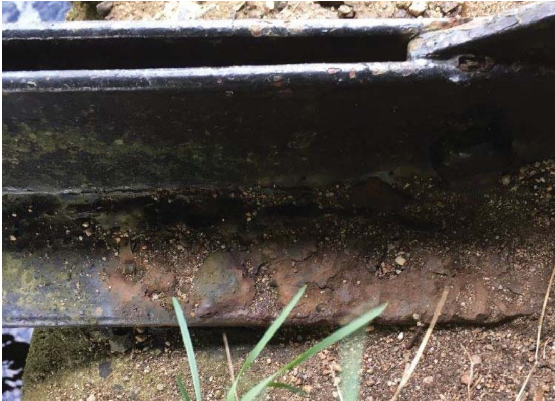
Photo 7 -SECTION LOSS AT NE TRUSS BEARING
