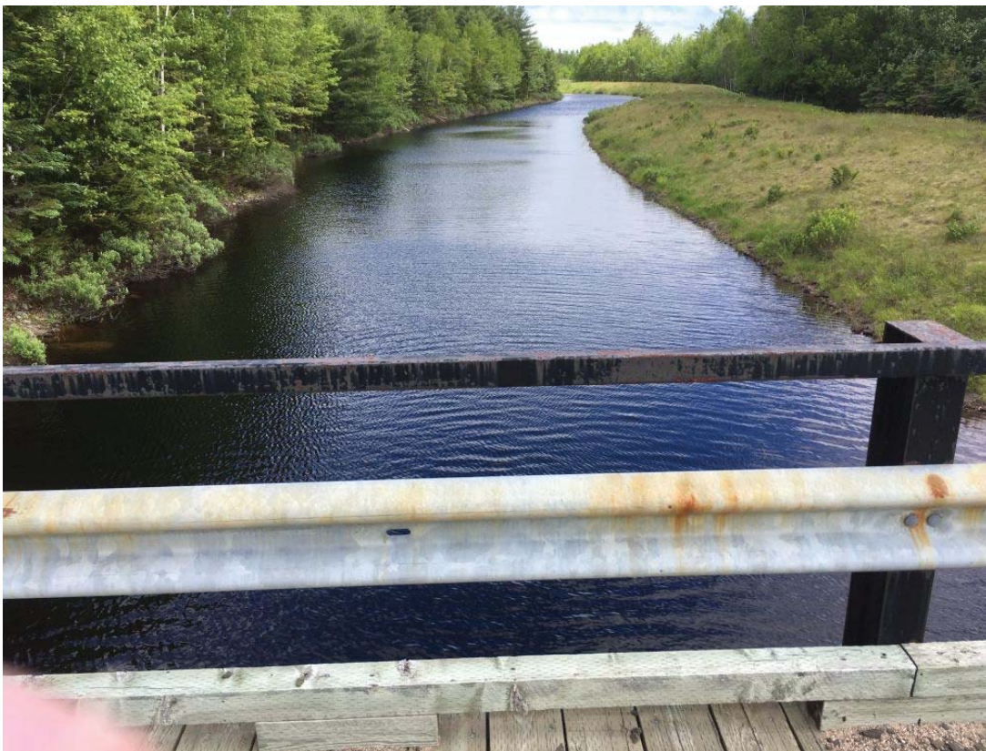
Photo 6 - ON BRIDGE LOOKING NORTH
