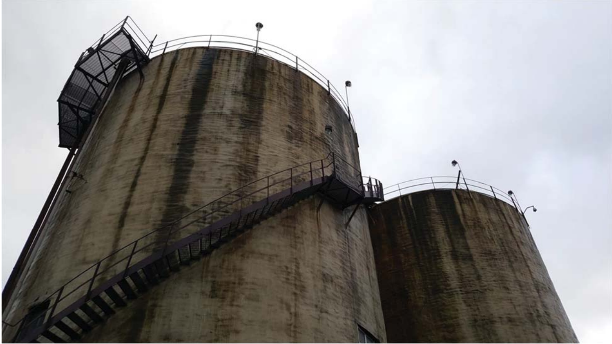
Photo 3: Showing a view mid-way up the stair system.
