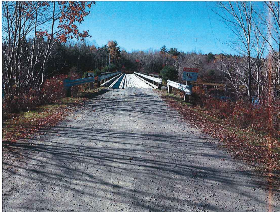
Photo 2 - LOOKING W ACROSS BRIDGE
