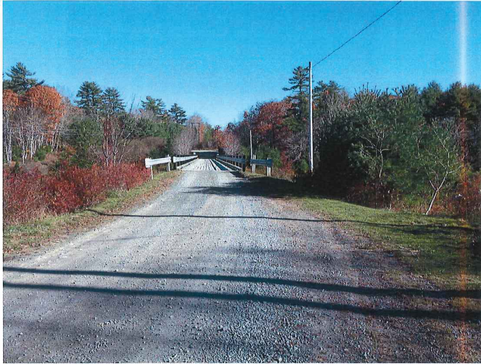
Photo 1 - LOOKING E ACROSS BRIDGE
