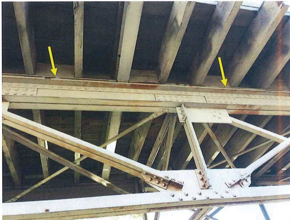
Photo 10 - TYPICAL UNDERSIDE OF DECK AND TRUSS. NOTE REINF TOP CHORD
