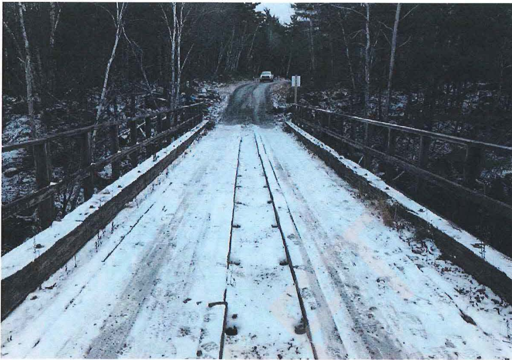
Photo No. 3 – Bridge Deck
