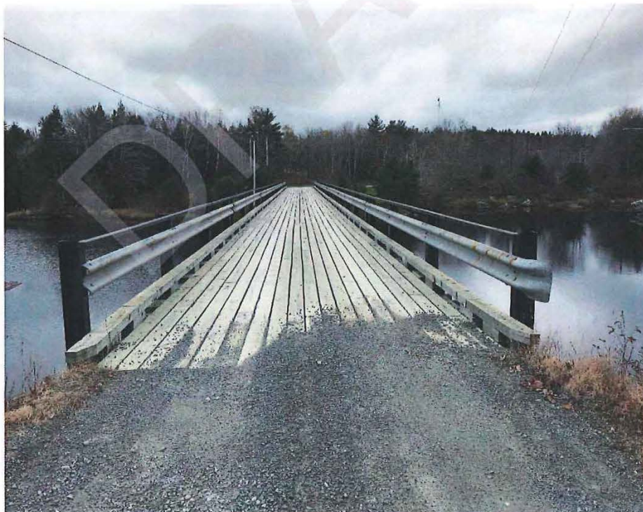
Photo No. 4 – Bridge 15 – Big Falls – Bridge Deck
