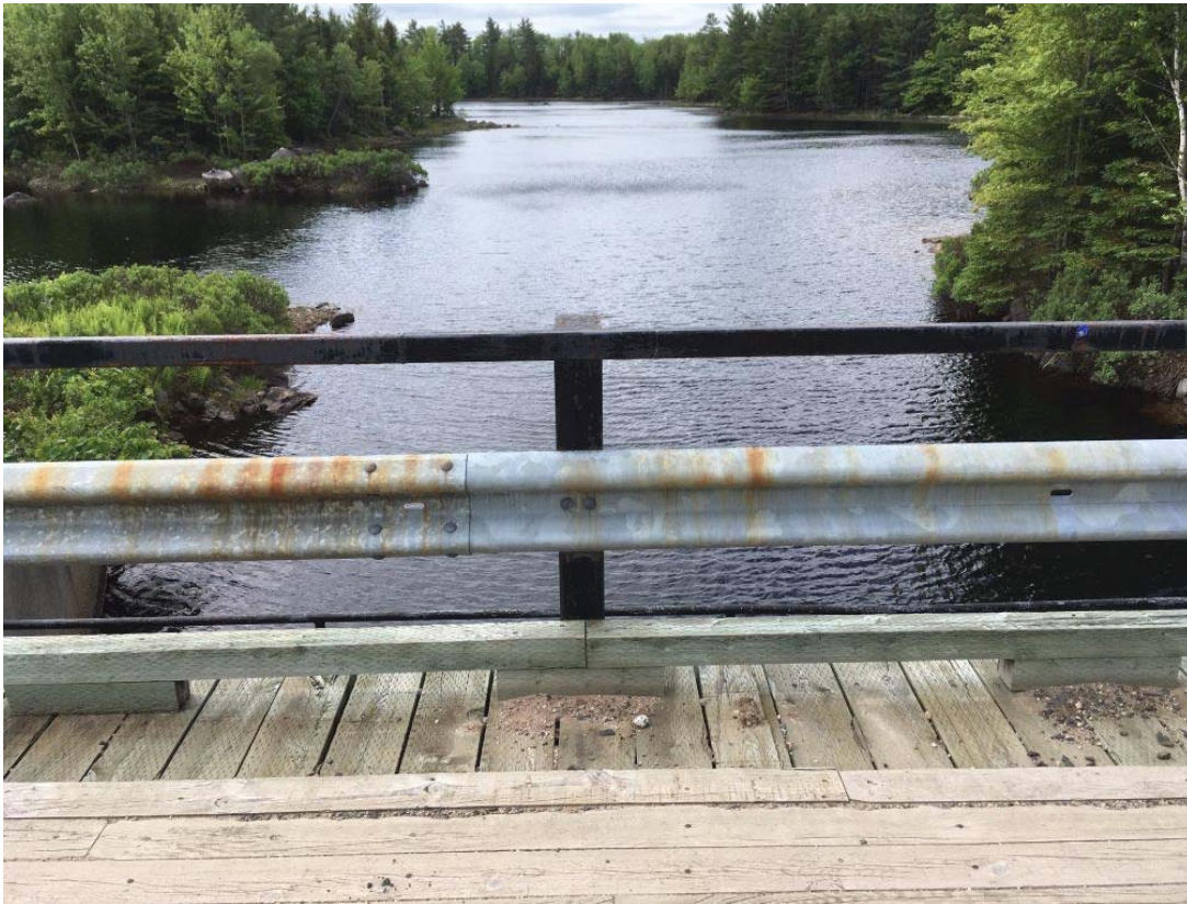
Photo 5 - ON BRIDGE LOOKING SOUTH
