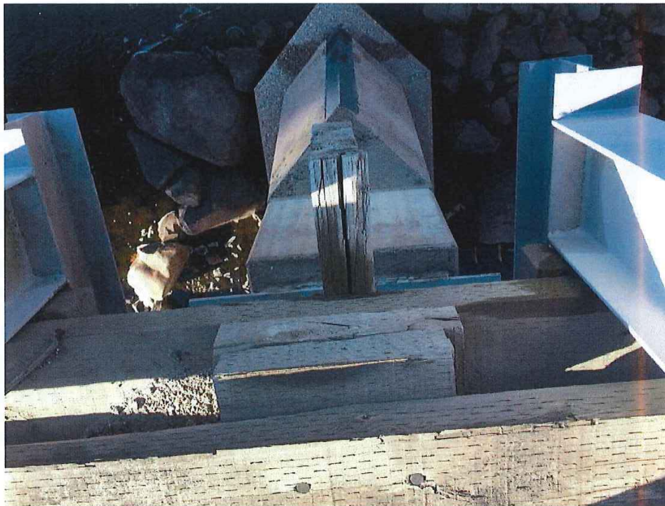
Photo 6 -LOOKING DOWN AT TYPICAL STRINGER AT PIER
