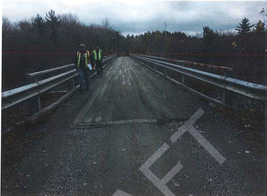
Photo No. 1 – Bridge 14 – Lower Lake Falls – Bridge Deck
