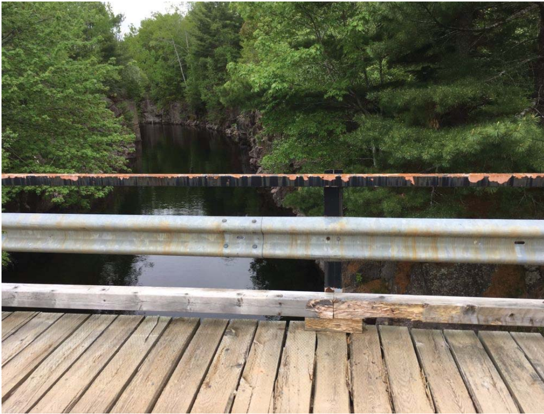
Photo 5 - ON BRIDGE LOOKING SOUTH (UP-STREAM)
