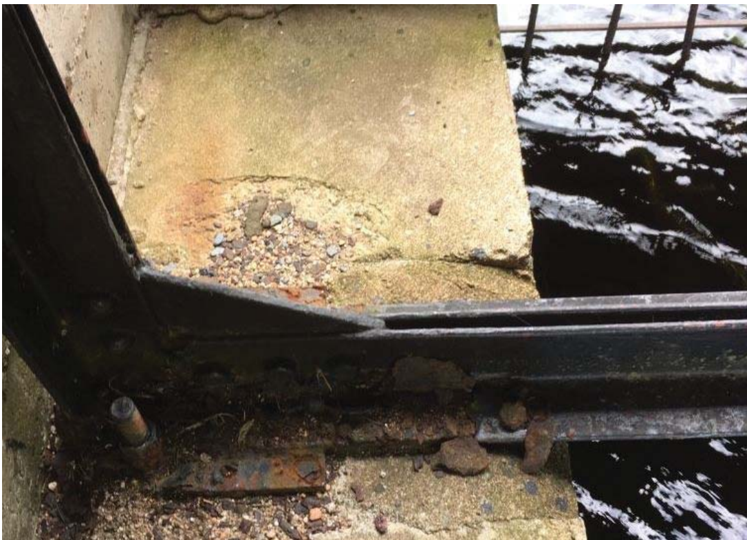
Photo 7 -SECTION LOSS AT NE TRUSS BEARING
