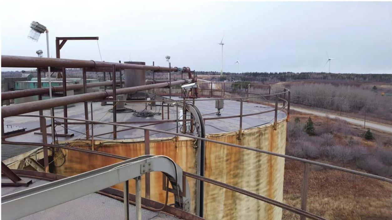
Photo 4: Showing a view of the Ash Silo Roof hand rail.
