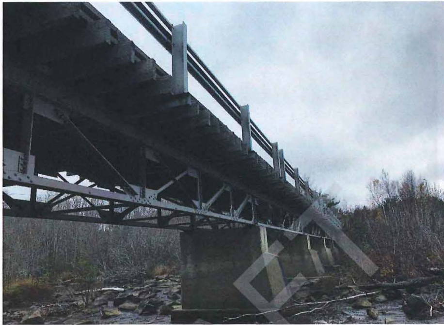
Photo No. 3 – Bridge 14 – Lower Lake Falls – Bridge Elevation
