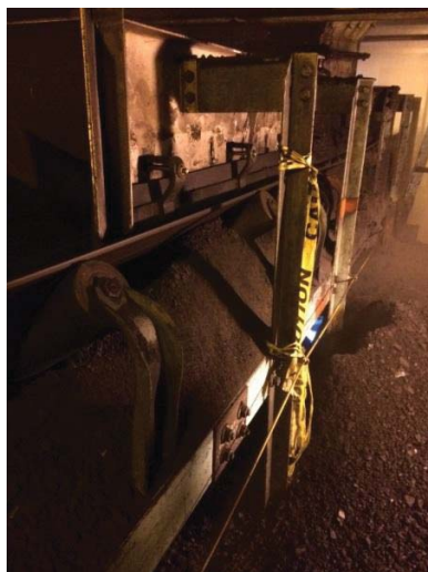
Existing Loading Zone at Trenton
