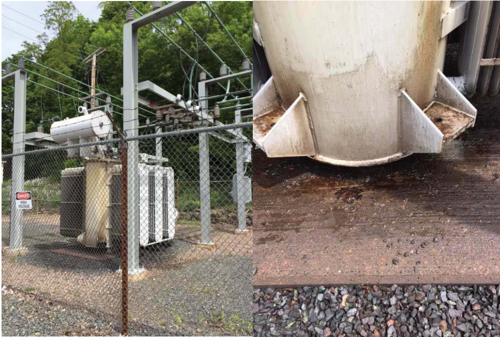
Figure 3 Photos of 61N-Provost St
