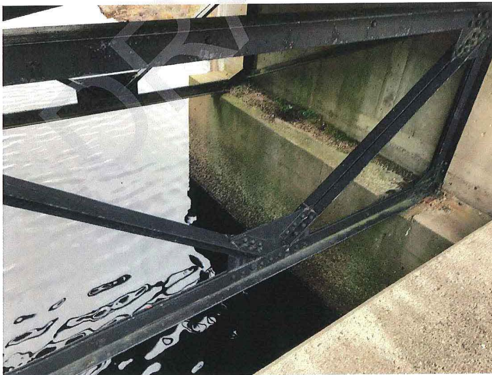
Photo No. 4 – Bearing Seat
