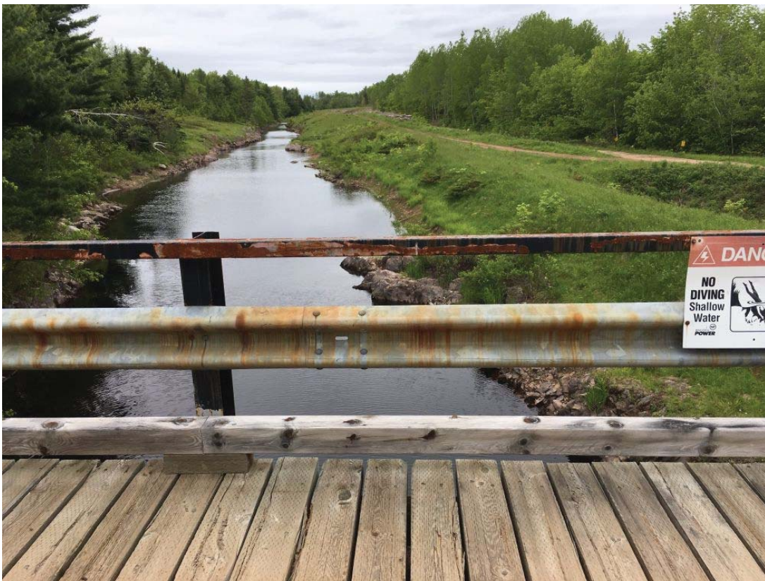
Photo 6 - ON BRIDGE LOOKING NORTH (DOWNSTREAM)
