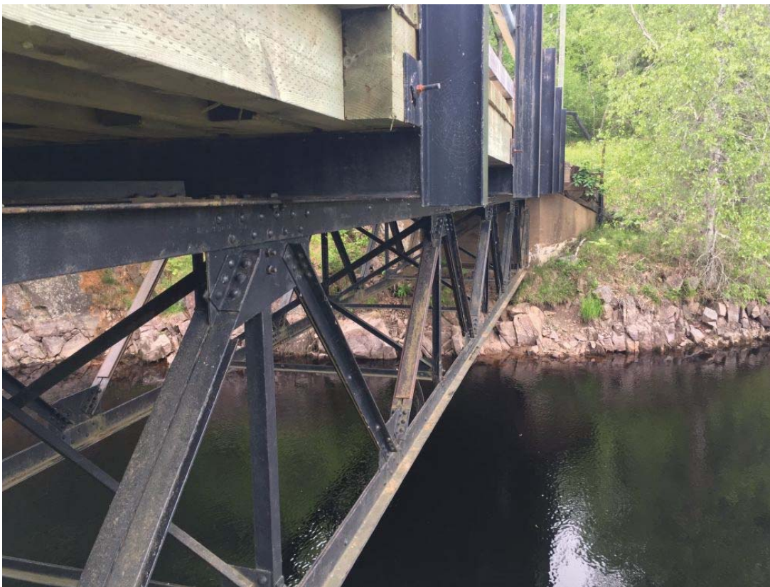
Photo 4 - PARTIAL N. ELEVATION SHOWING REINFORCED TRUSS MEMBERS
