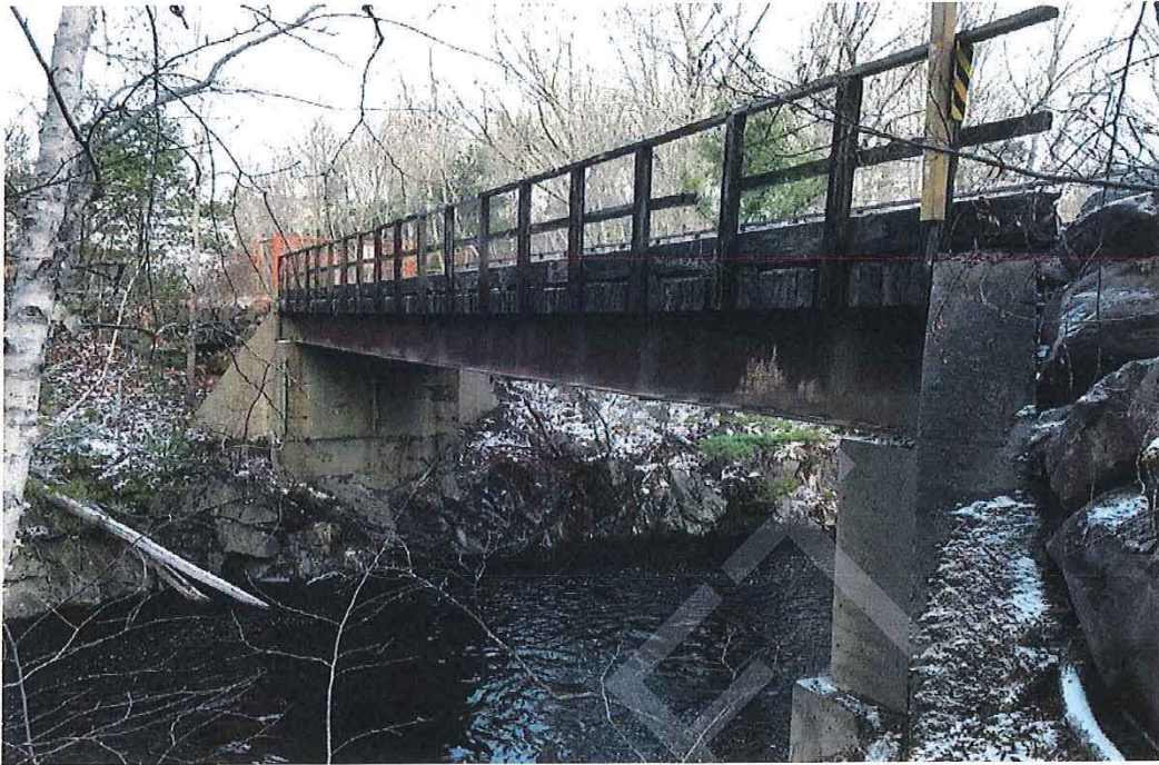
Photo No. 5 – Bridge Elevation
