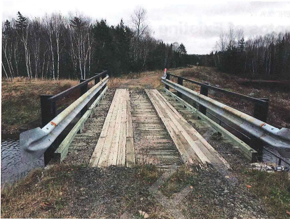
Photo No. 1 – Bridge Superstructure
