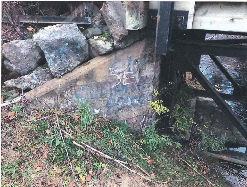
Photo No. 2 – Existing abutment wing wall.
