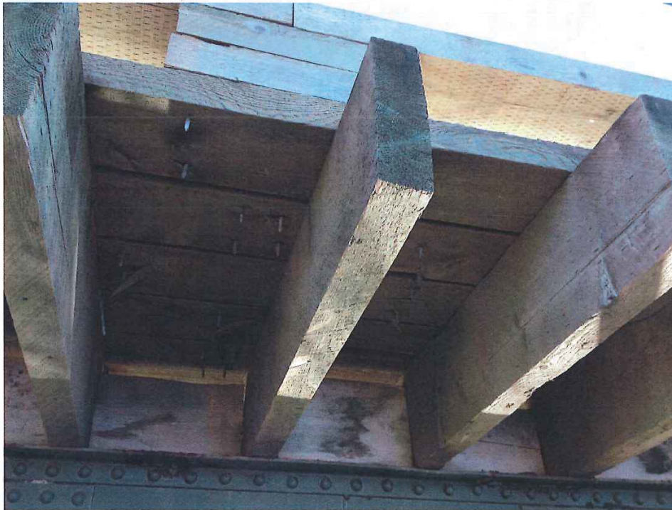
Photo 12 - TYPICAL UNDERSIDE OF DECK/STRINGERS
