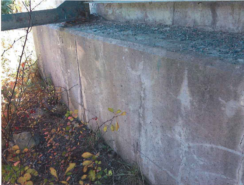
Photo 19 - W BREASTWALL/BEARING SEAT
