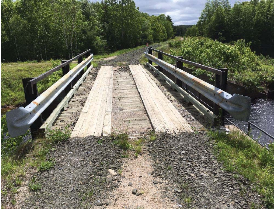
Photo 1 - APPROACH LOOKING EAST
