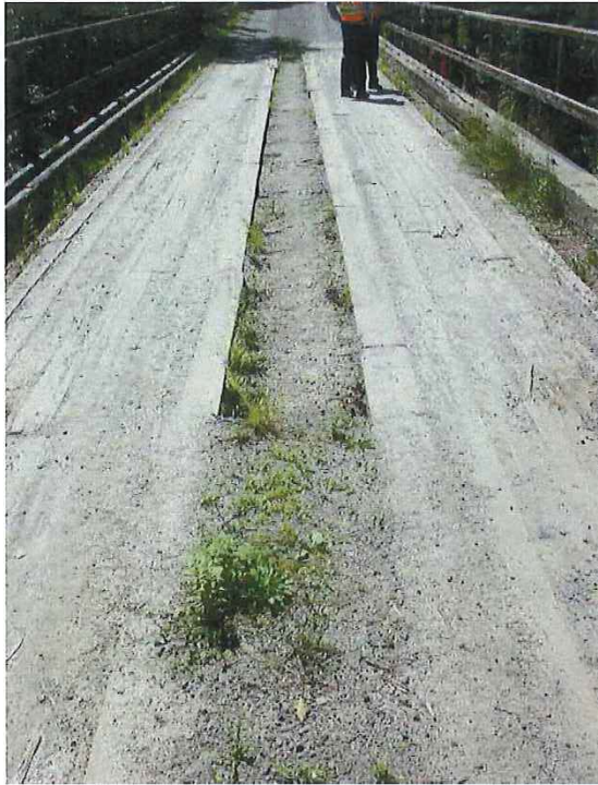
Photo 5 - Wearing Surface looking south
