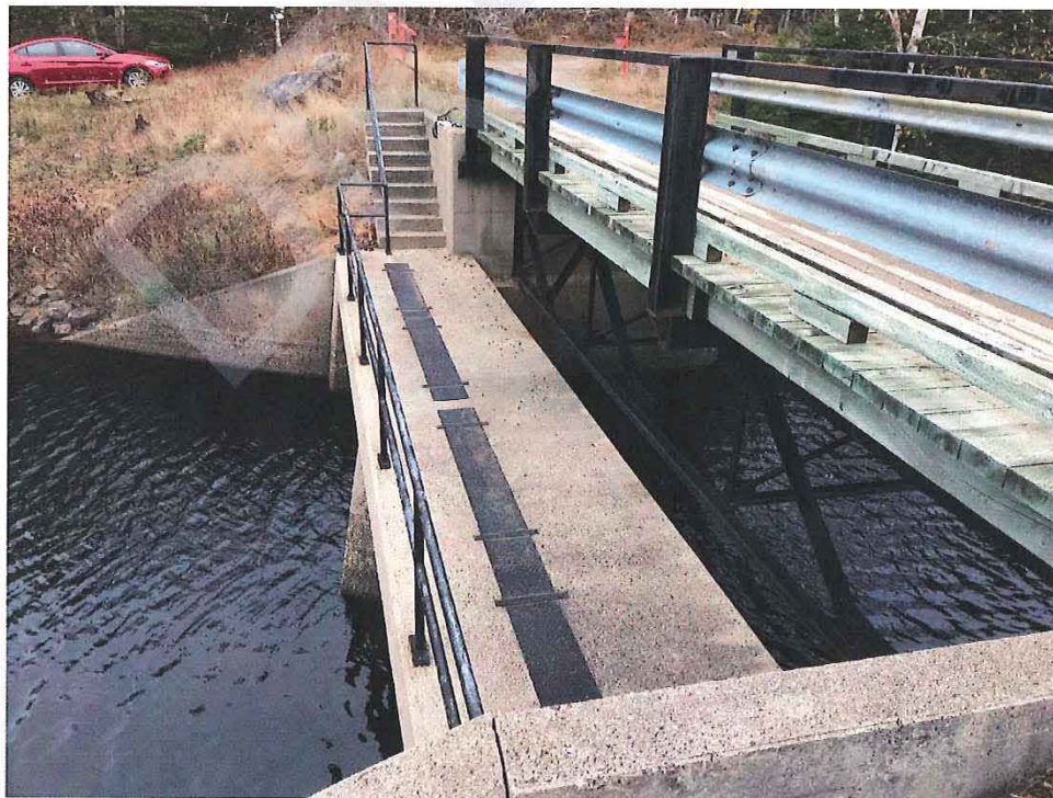
Photo No. 2 – Bridge Elevation
