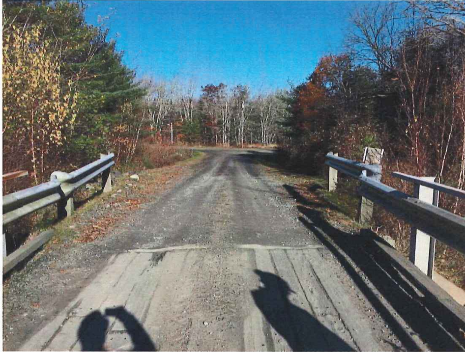
Photo 7 -LOOKING N FROM BRIDGE
