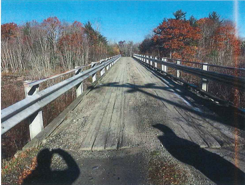
Photo 1 -LOOKING N ACROSS BRIDGE
