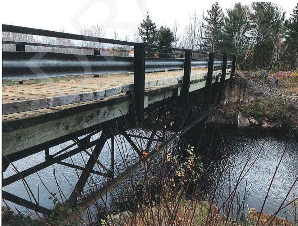
Photo No. 4 – Existing superstructure elevation.
