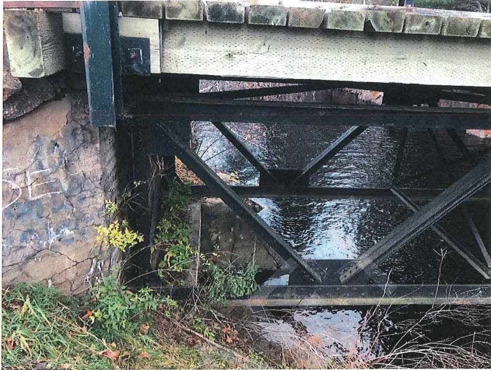
Photo No. 3 – Existing abutment wing wall.
