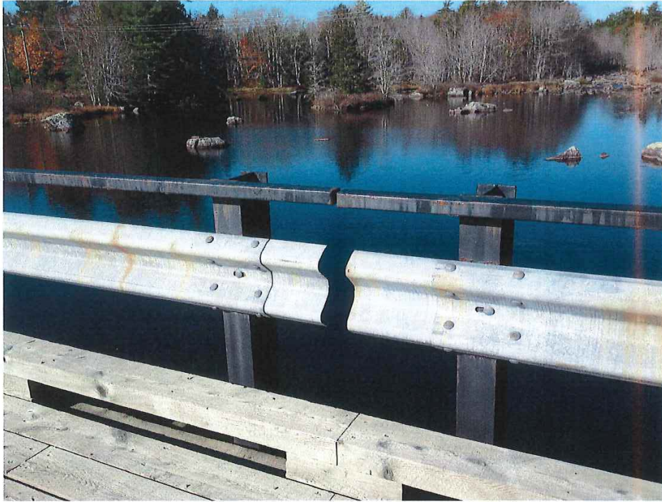
Photo 5 - TYPICAL "EXPANSION JOIT" BETWEEN TRUSSES
