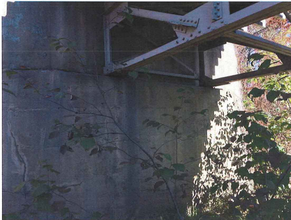
Photo 8 - LOOKING AT N ABUTMENT
