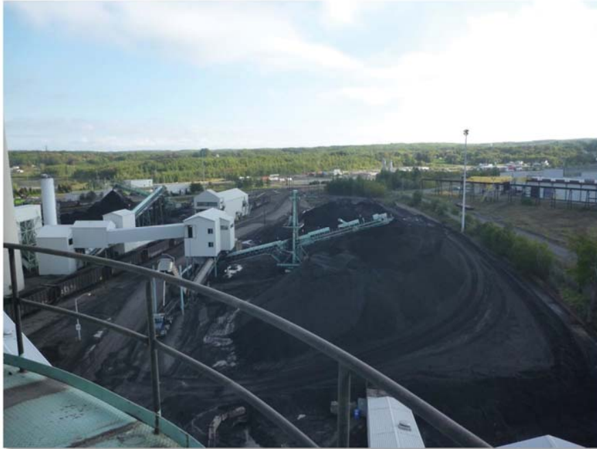
Trenton Coal Storage Pile
