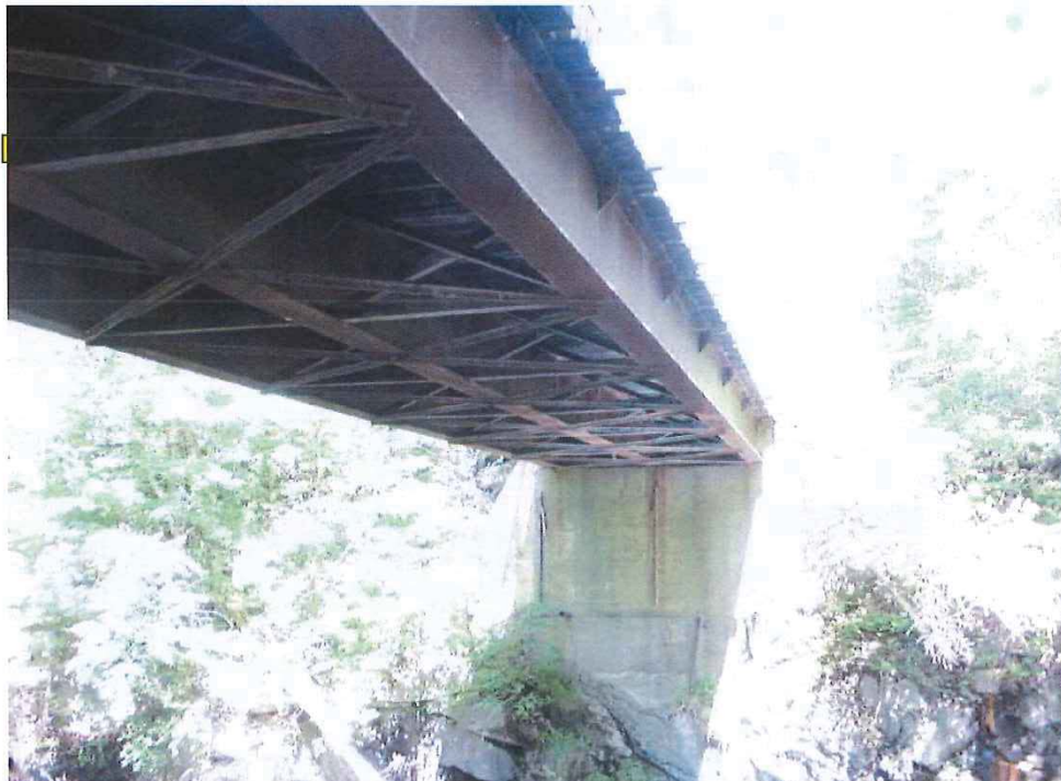
Photo 8 - Girders and Cross Beams - Looking North
