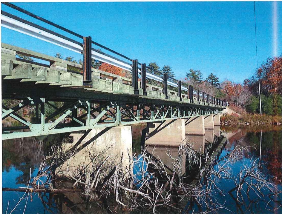
Photo 22 - LOOKING AT S SIDE OF BRIDGE
