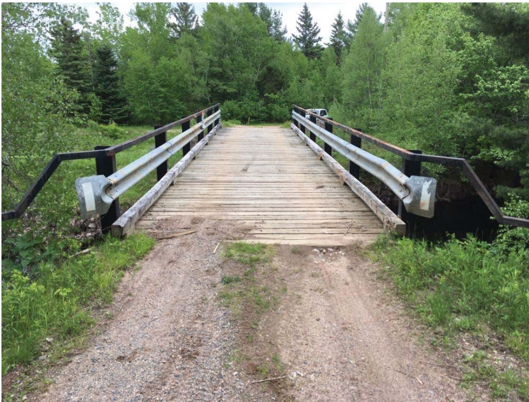
Photo 2 - APPROACH LOOKING EAST
