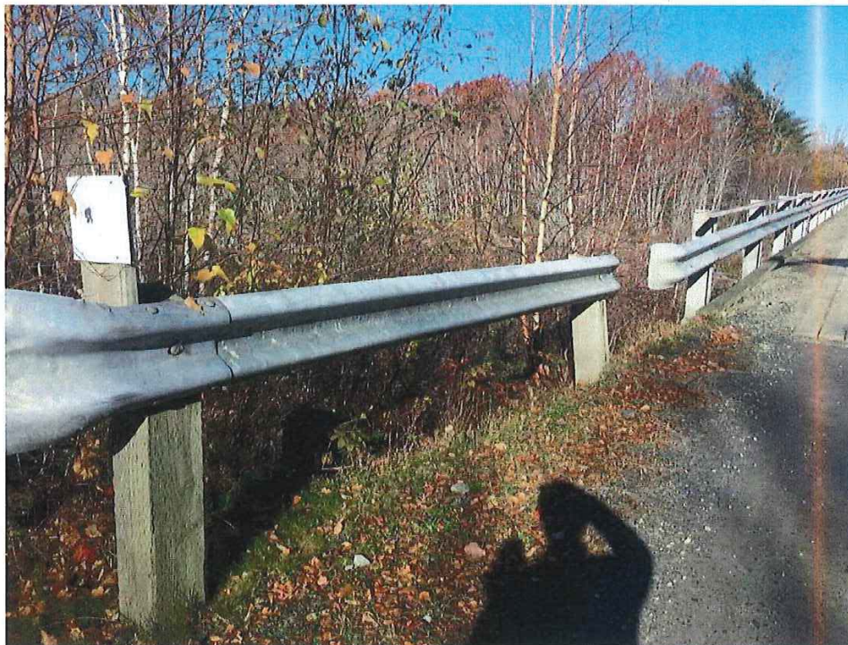
Photo 2 - SW APPROACH RAIL
