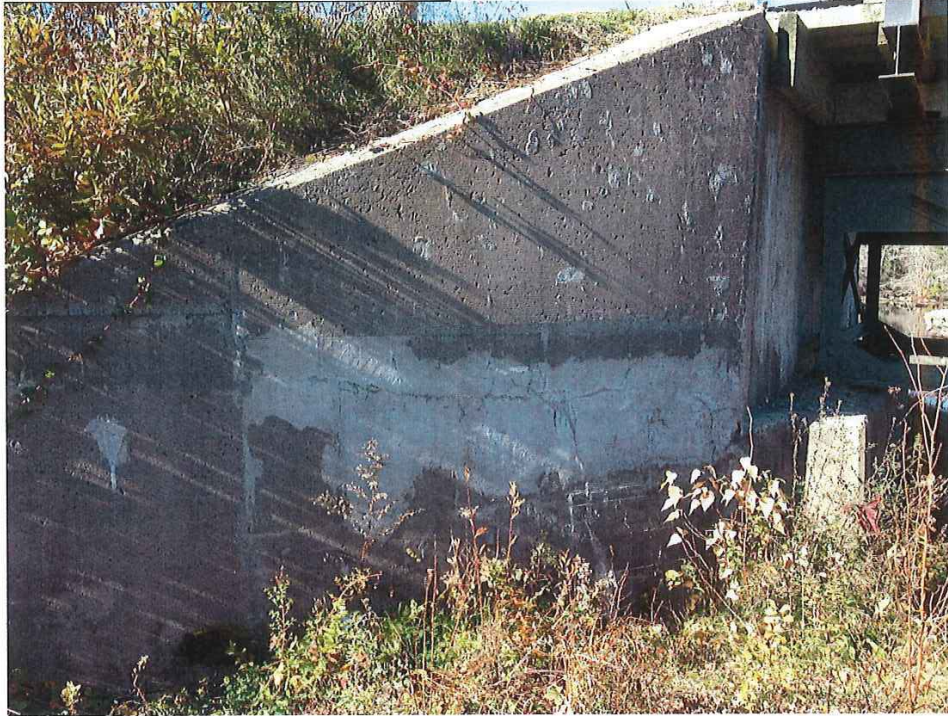
Photo 21 - SW WINGWALL REPAIRED
