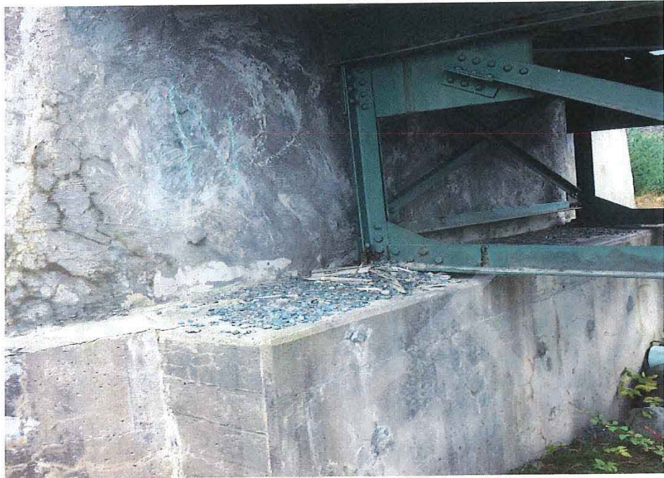
Photo No. 5 – Bridge 15 – Big Falls Bridge Abutment
