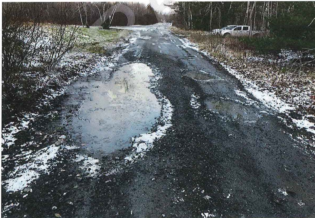
Photo No.2 – Bridge Approach
