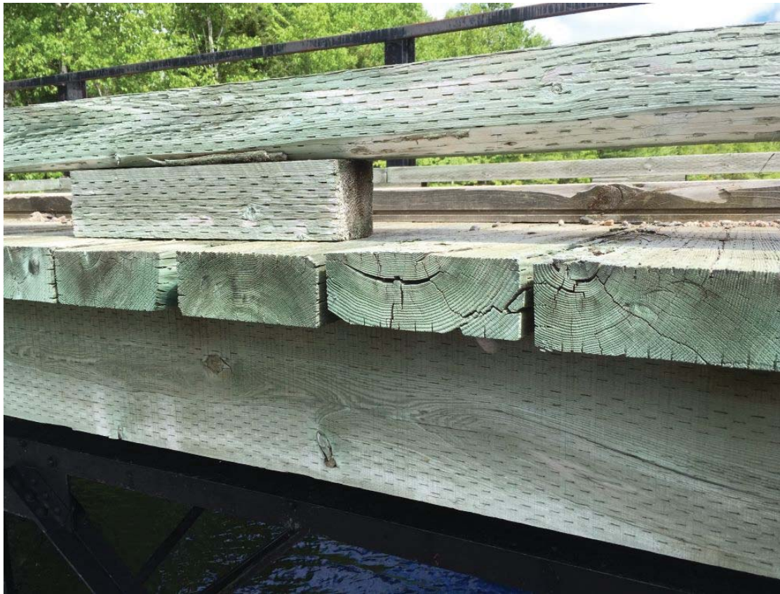
Photo 15 - TYPICAL CHECKING AT ENDS OF DECK SHEATHING
