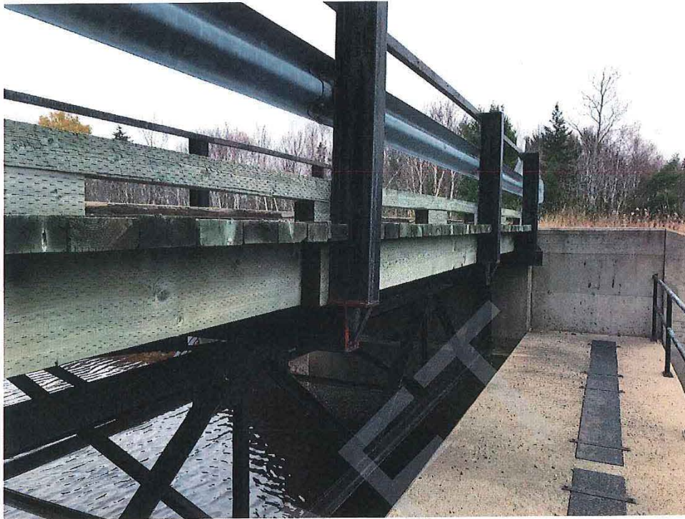
Photo No. 3 – Bridge Partial Elevation
