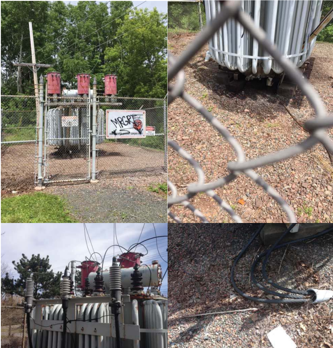
Figure 6 Photos of 532N-Elm St
