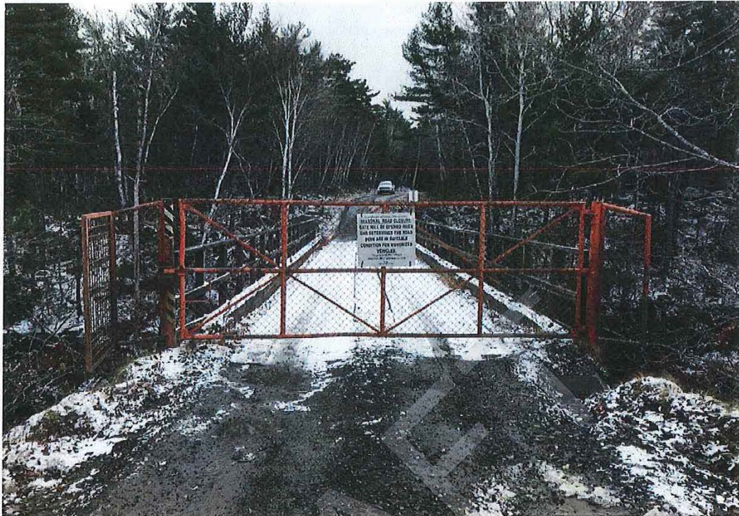
Photo No. 1 – Bridge Deck and Gate
