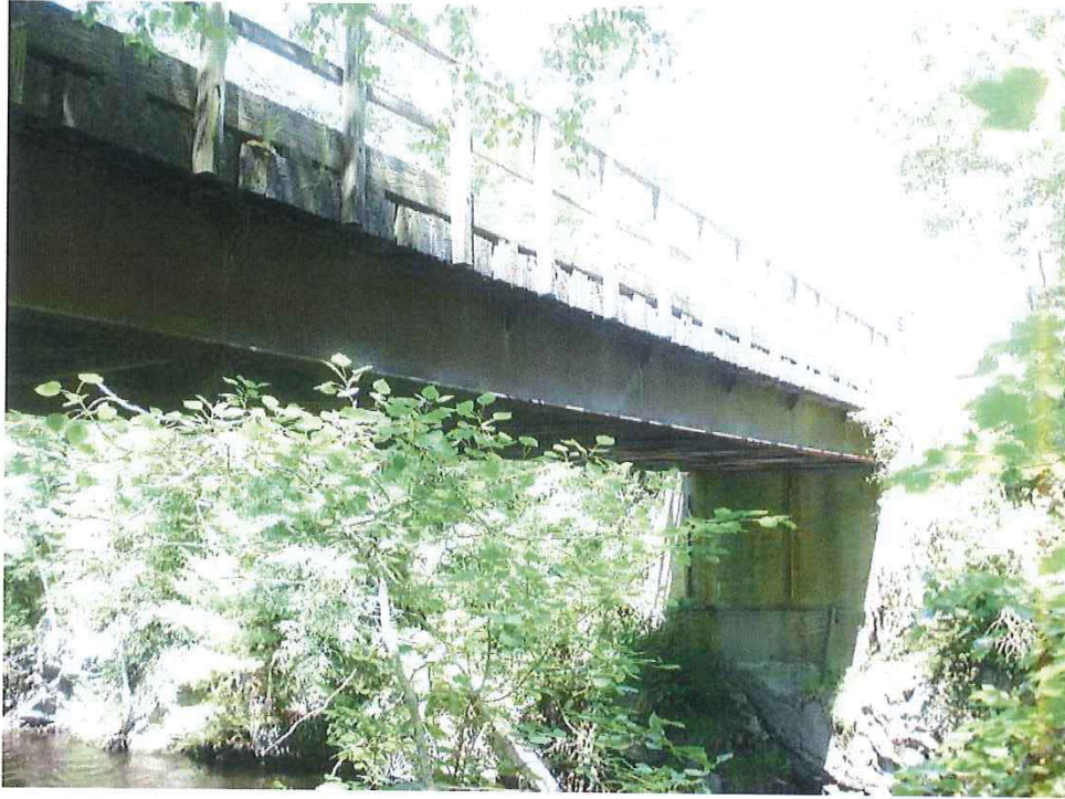
Photo 9 - Girders and Abutment - looking north
