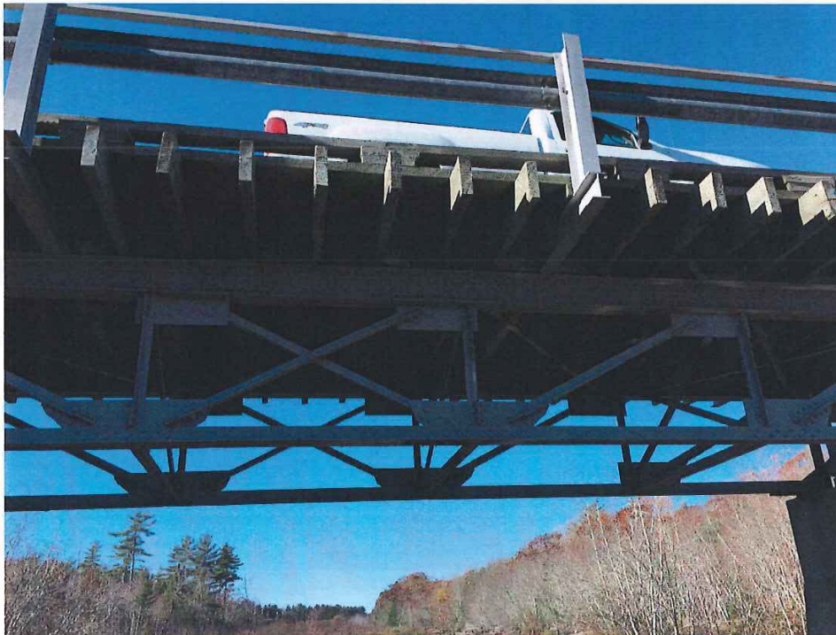
Photo 16 - TYPICAL UNDERSIDE OF TRUSS
