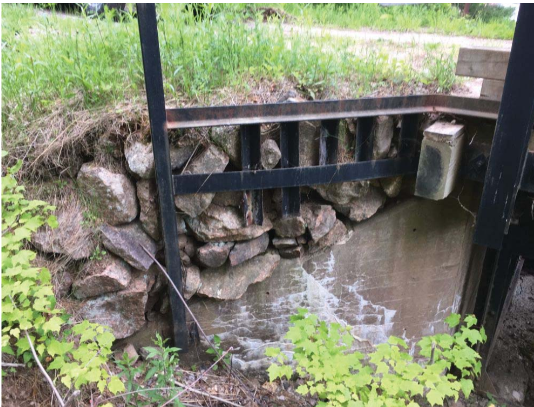
Photo 18 - TYPICAL WINGWALL EXTENSION
