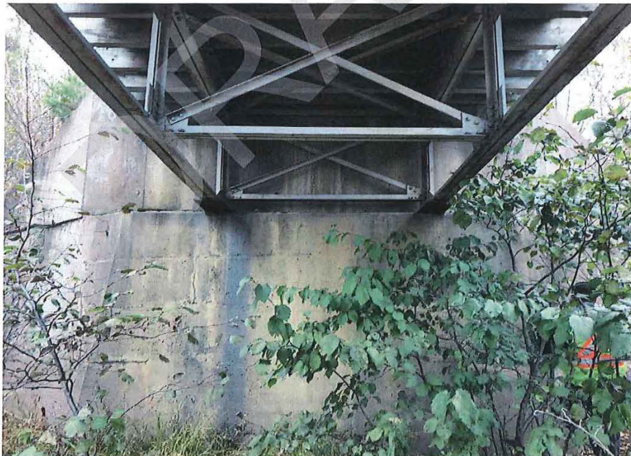
Photo No. 2 – Bridge 14 – Lower Lake Falls – Bridge Abutment
