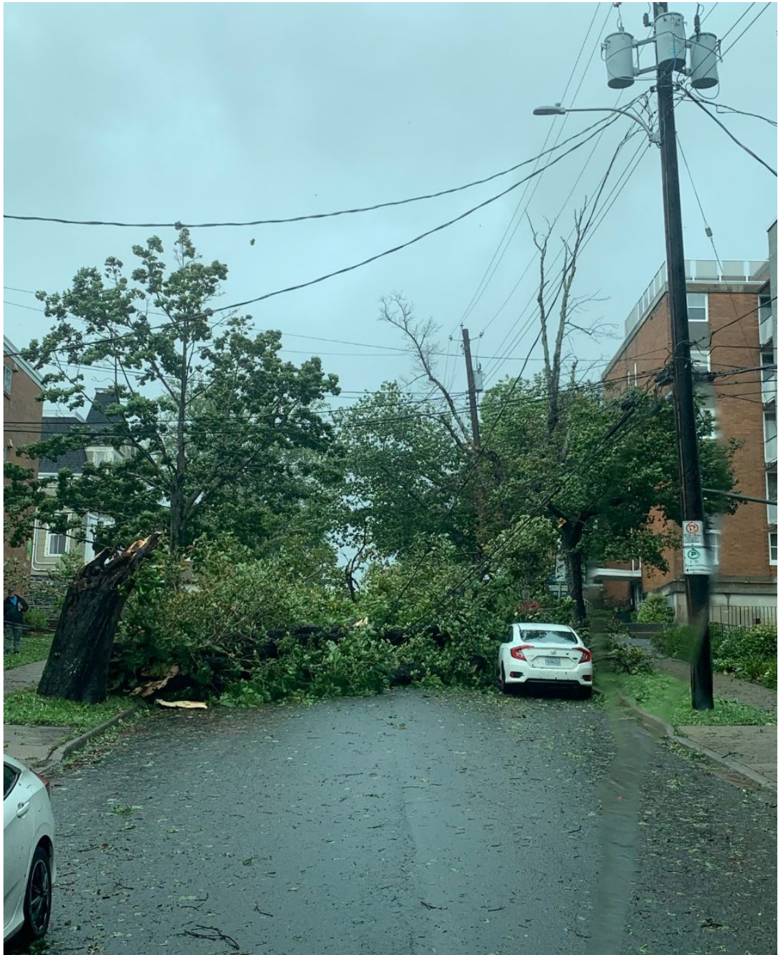
Figure 67 - Power Line Damage from Post Tropical Storm Lee
